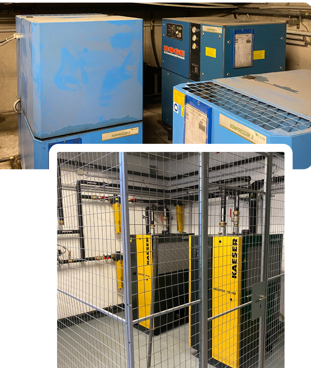
Figure 2: Old compressors (top) are replaced by a new compressor system with heat recovery (bottom) to allow for electric power and thermal energy saving. (Source: GW St. Pölten)
