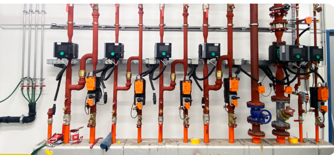
Figure 1: The new distribution system is a fully hydronic balanced system using pressure-independent control valves that also allows the measurement and control of energy flows. (Source: GW St. Pölten)
